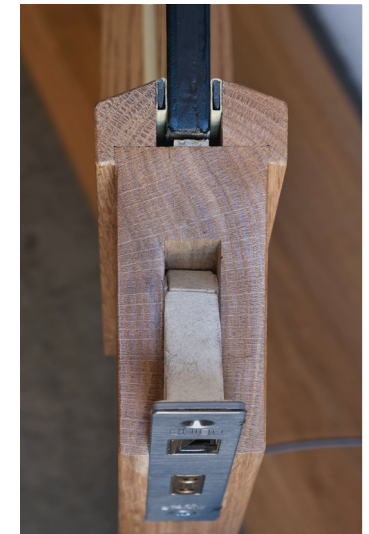
Intumescent around lock
